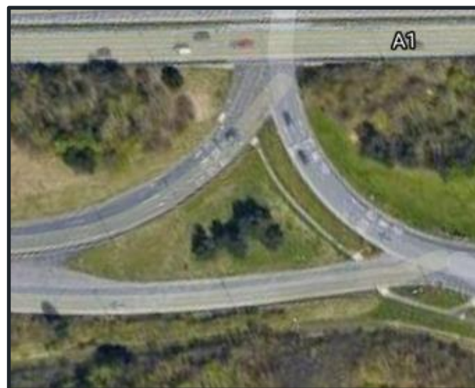
Figure 14: Outfall 5 Aerial View (Google)
