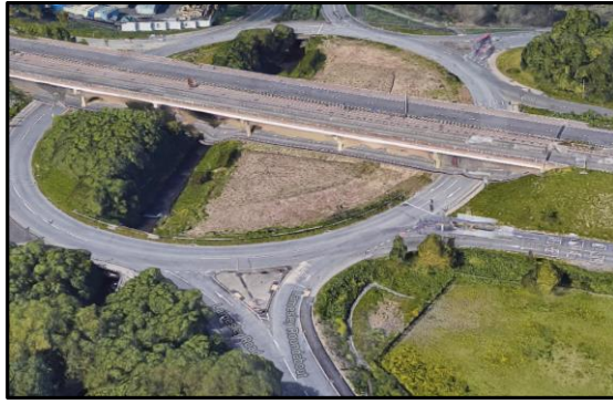
Figure 38: Outfall 13 Street View (Google)
