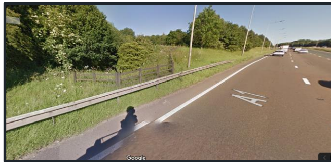
Figure 21: Outfall 7 Street View (Google)
