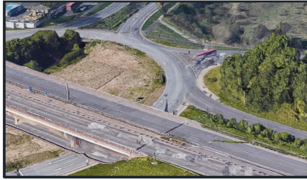
Figure 32: Outfall 11 Street View (Google)
