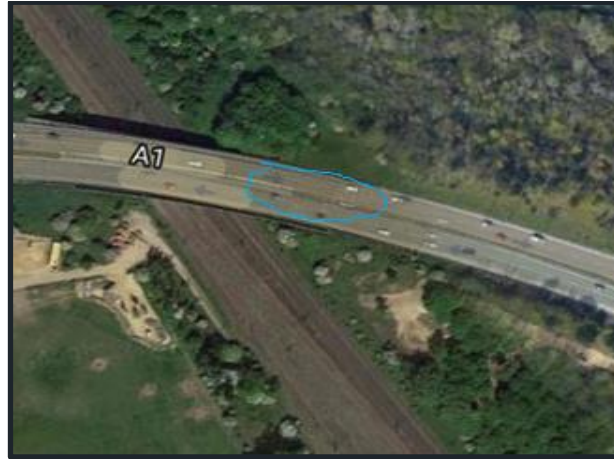
Figure 25: Outfall 8 Aerial View (Google)
