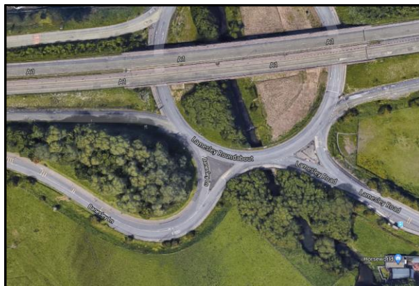
Figure 37: Outfall 13 Aerial View (Google)
