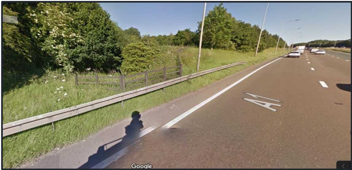
Figure 23: Outfall 7a (VS1 & VS2) Street View (Google)
