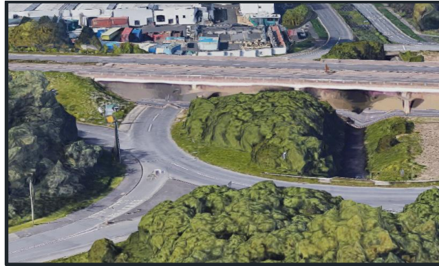
Figure 35: Outfall 12 Street View (Google)
