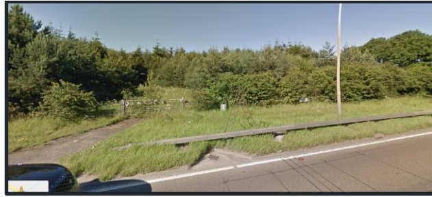
Figure 12: Outfall 4 Street View (Google)
